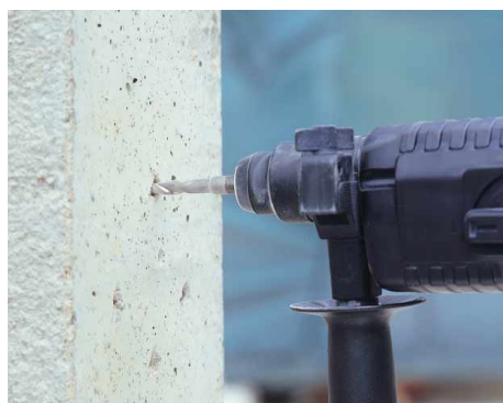
Drill the hole for the anchor with the hammer drill.
