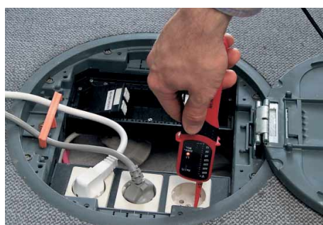
One-pole phase test.
