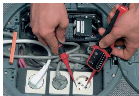
Residual current triggering (up to 30 mA).
