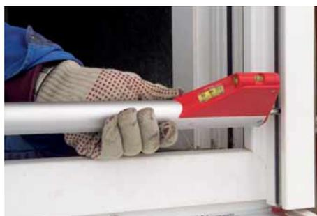
For measuring in roller shutter guides
