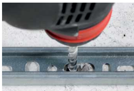
Fastening with plastic frame anchor W-UR for C-rail 26/18
