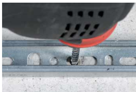
Fastening with mounting rail screw type MS for C-rail 26/18
