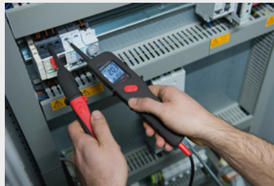
Voltage test DC
